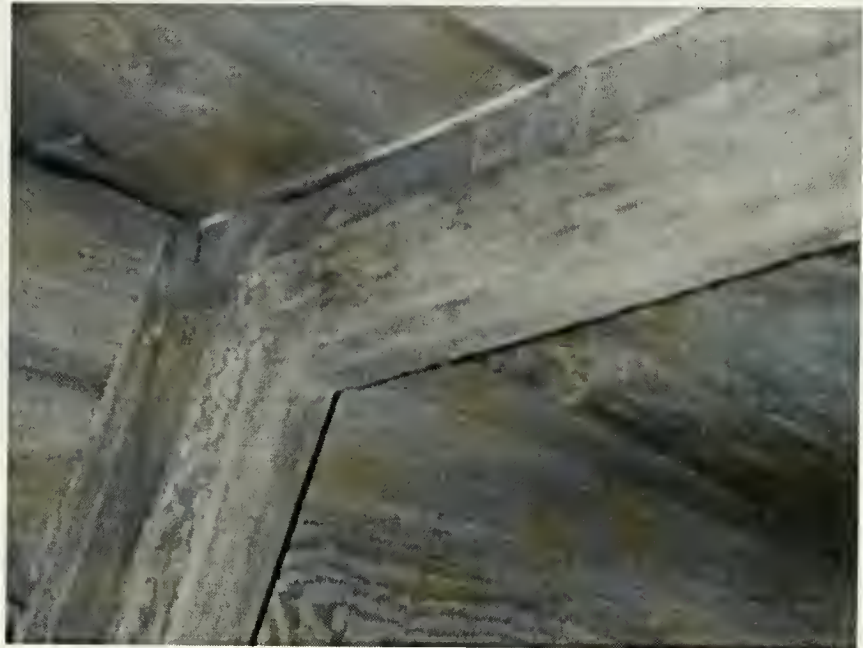
Figure 8 Original Rafter in Center Section of Main House, 2002
